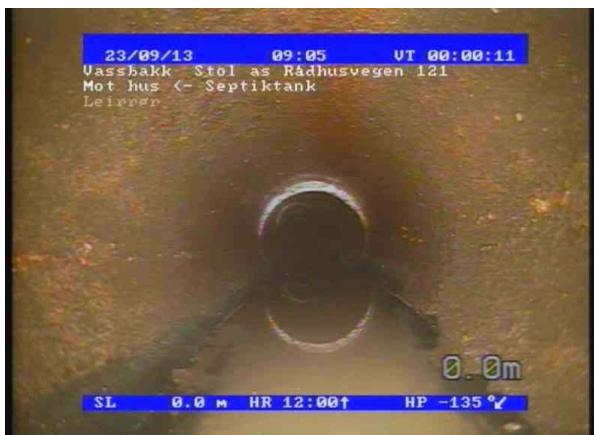
13.09.2023 08_56_59_0f6fcddc-caca-4c73-87b7-860e698c6fc7_20230914_080410_327.jpg, 00:00:11, 0.00 Vannivå, 5%, start
