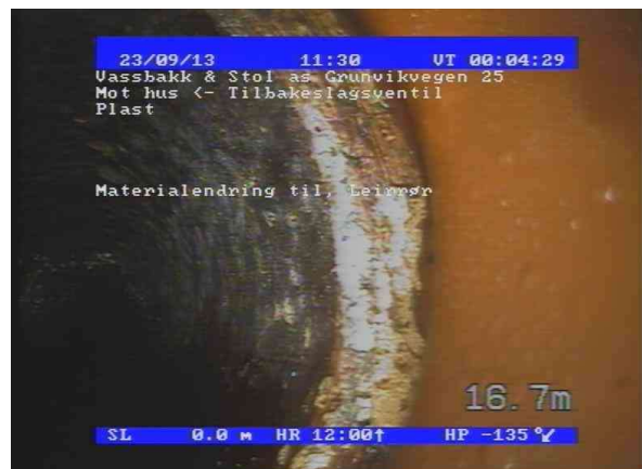
13.09.2023 10_47_59_1d496805-7de6-4984-ac0e-dea97bd88ee1_20230 913_112323_597.jpg, 00:04:24, 16.70 Materialendring til, Leirrør
