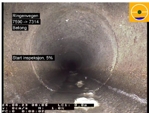
24.08.2023 080713_7314_7590_24082023_080913_002.jpg, 00:00:00, 0.00m Start inspeksjon, 5%
